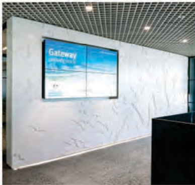
Column & Wall Cladding
